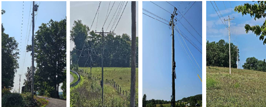
Standardsville Area Completed fiber installation on REC poles
